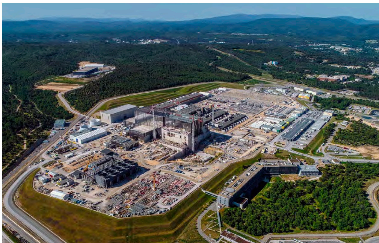
Fot. 6. Obszar budowy reaktora ITER, stan na 27 maja 2020. (fot. ITER Organization, EJF Riche) Photo 6. The ITER reactor construction area, as of May 27, 2020 (Photo: ITER Organization, EJF Riche)
